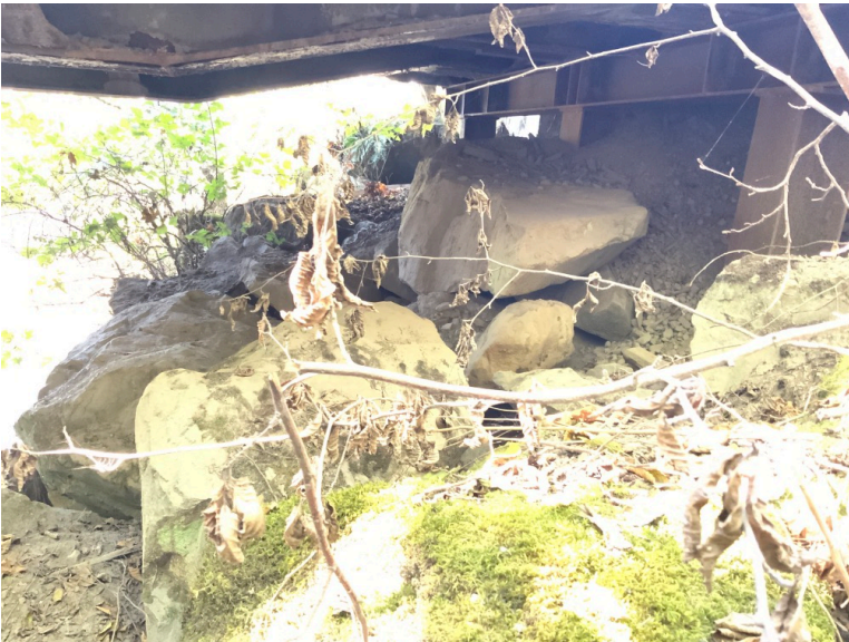
Right Bank Abutment when facing downstream
