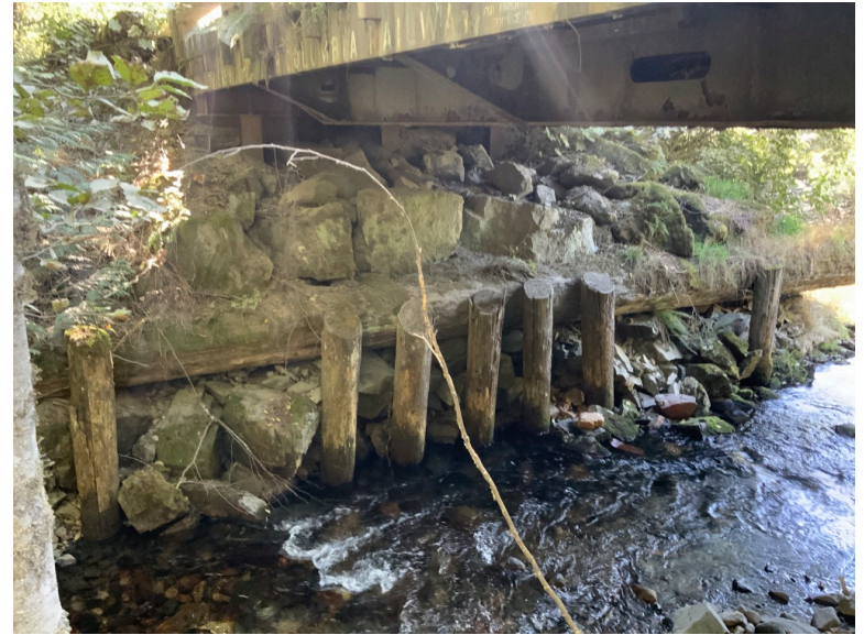
Left Bank Abutment when facing downstream
